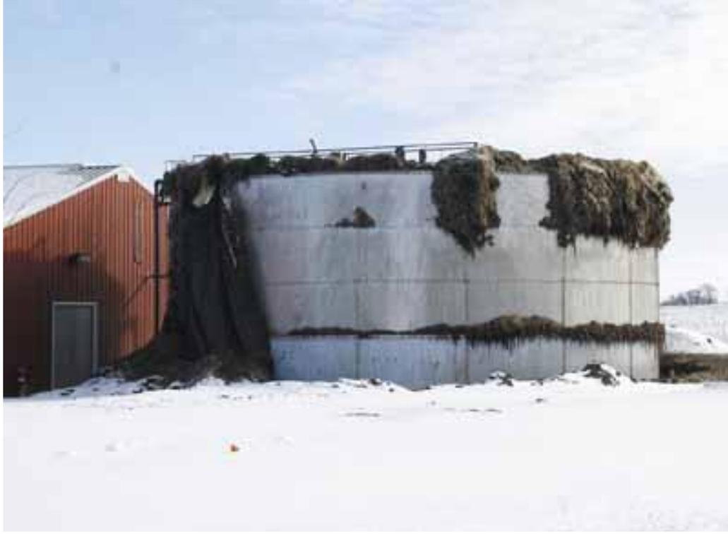
**Waste treatment tank at Cavel ruptures and foams over, March 2007.**
